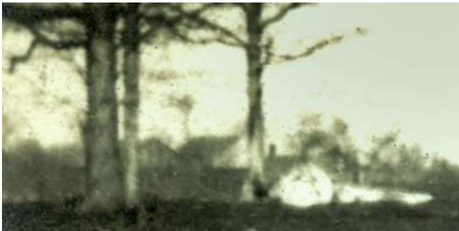
Figure 86 The buildings of John Cannon and his neighbour across the street at the end of Golf Course Lane appear in this greatly enlarged detail from Mary Vrooman's photograph of Bennett, Herrington, and Hall.
