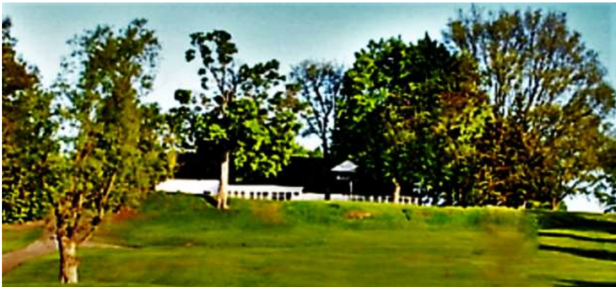
Figure 103 Trees unpruned in eighty years obscure the part of the clubhouse representing the original clubhouse.
