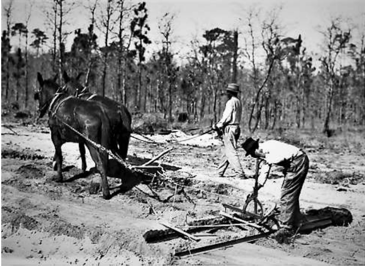
Figure 27 Muleskinners deploy a "Railroad Plow" or "Sturdy Plow" to smooth the surface of the soli piled on the green site.
