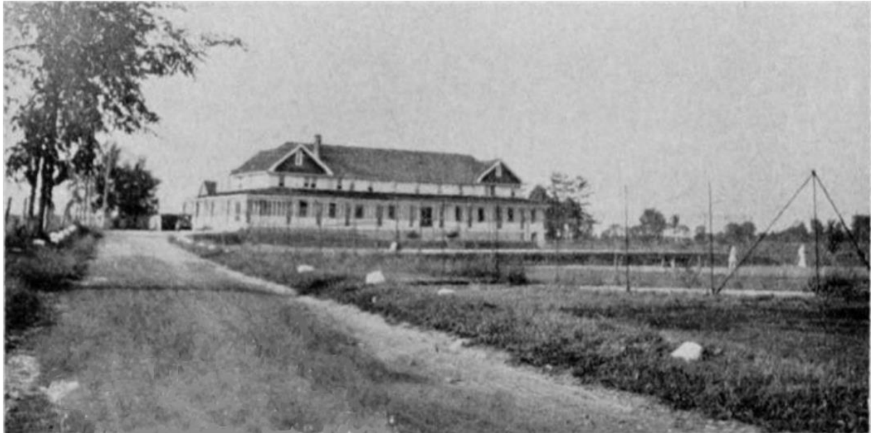
Figure 66 Highlea Tennis and Country Club, Aylmer Road (opposite the grounds of the Chaudière Golf Club), circa 1928. This clubhouse is marked on the map in Figure #3 above.
