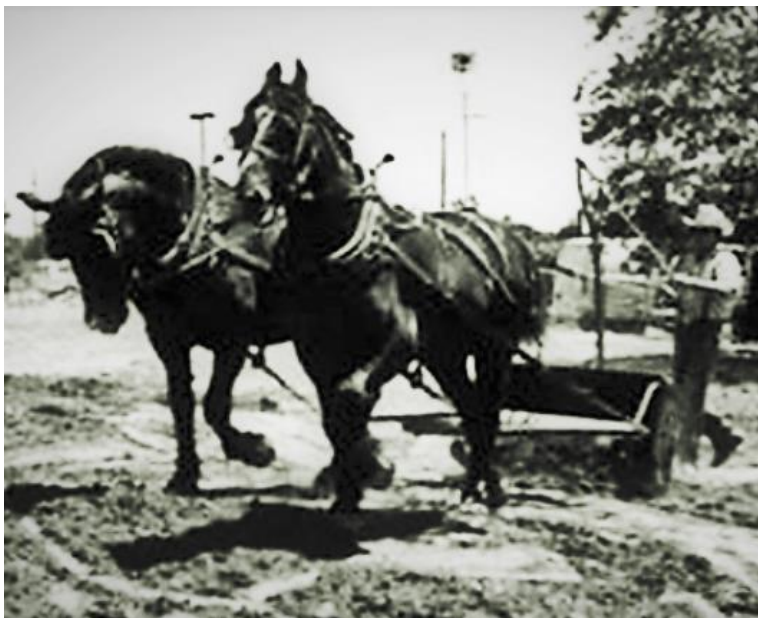
Figure 54 The operator has tilted the handle of the Fresno Scraper upright to empty the bucket. He holds a rope attached to the handle to pull it back down when the bucket is empty.
