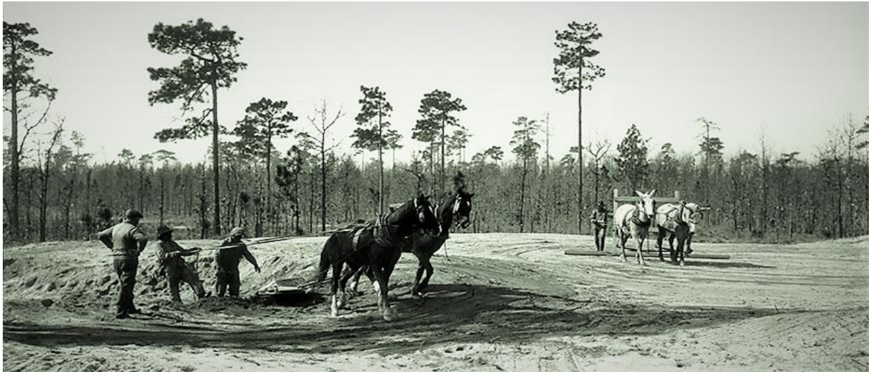
Figure 55 Fresno Scraper and Railway Plow operating in concert during green construction.
