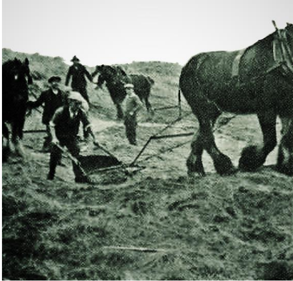
Figure 53 Fresno Scraper teams building bunkers and greens. Harry S. Colt and C.H. Alison, Some Essays on Golf Course Architecture (London: Country Life, 1920).
