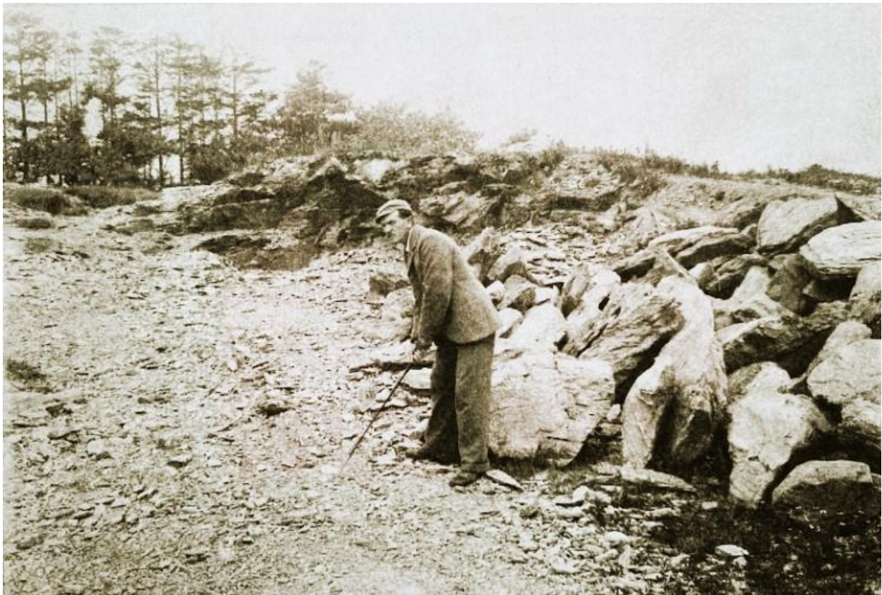
Figure 41 I believe that this photograph shows Willie Davis posing in the quarry of the hole called "Quarry" at the Newport Golf Club. The hole retained the name "Quarry" on both the nine-hole layout begun in 1894 and the eighteen-hole layout opened in 1897. Photo courtesy of Susan Martensen. The latter is the great-granddaughter of Willie Davis.
