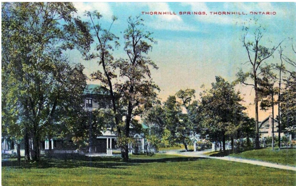
Figure 61 The Hawthorn Springs Residence depicted here became the clubhouse of the Thornhill Golf Club when the latter purchased the Hawthorn Mineral Springs and Residence Resort in 1922. The old clubhouse was demolished in 1963.
