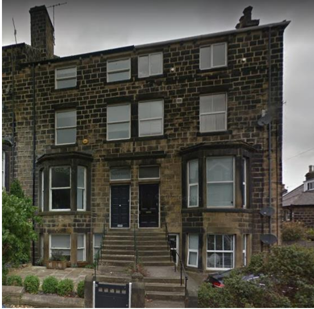
Figure 3 19 Tivoli Place, Ilkley, Yorkshire (left side of the house)
